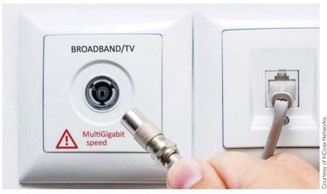
Brownfield MDU buildings have existing coaxial cabling or telephone lines that offer a multi-gigabit alternative to laying fiber directly to the premises.
